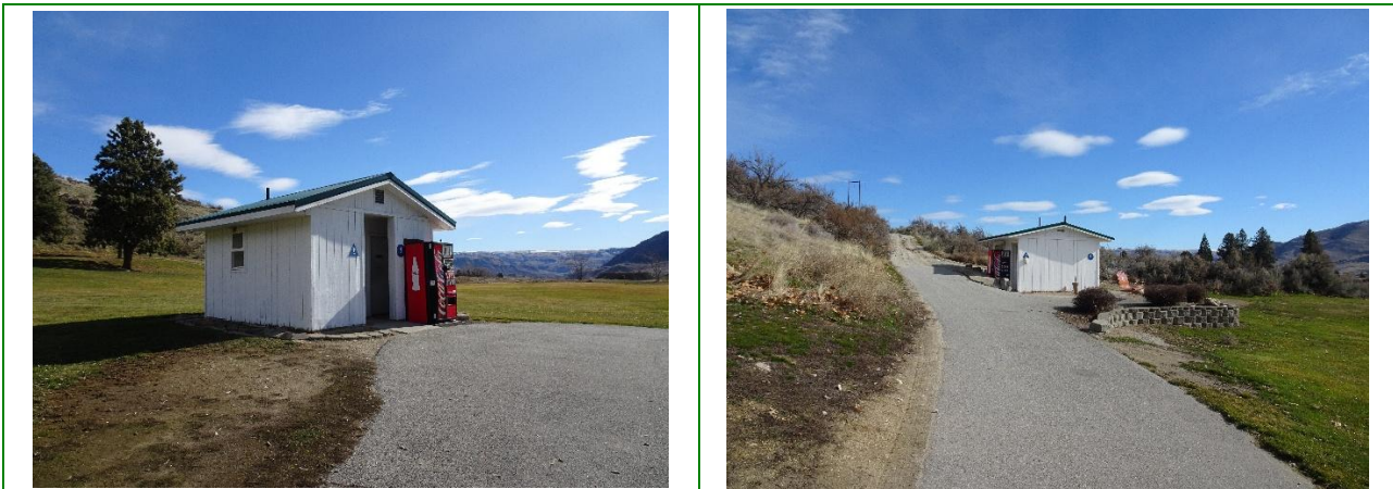
Images of on-course services at LCGC in 2026 that includes a beverage vending machine at each station (soft drinks only), potentially impacting the demand for beverage service from on-course staff using a vending cart (can allow beer/alcohol on vending cart).
