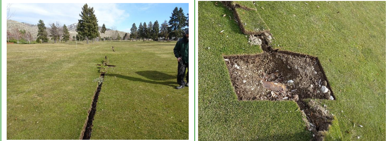
Images of ongoing drainage enhancements on hole #17 in February 2026.
