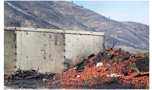
Chelan Complex fire effects on Chelan Fruit in Industrial Area Good Fruit Grower Magazine, November 17, 2015
